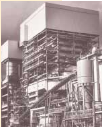
Photo courtesy of Western Power
