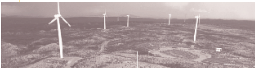
Photo courtesy of Western Power
