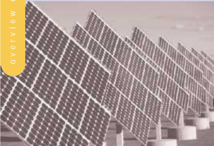
Photo courtesy of Western Power
