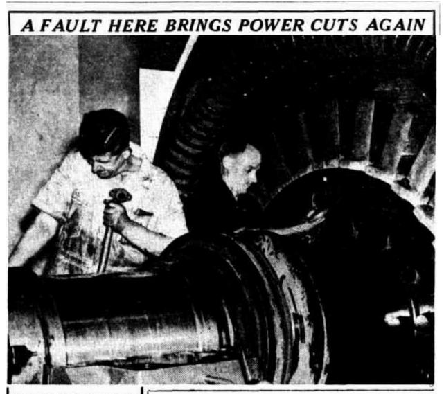
State Electricity Commission men working yesterday on the dismantling of the frequency changer at the East Perth power station in which a fault developed early yesterday morning, plunging Perth in darkness during an electrical storm. The fault prevents the S0-cycle electricity from the South Fremantle power station being converted to 40cycle frequency, which is used throughout most of the metropolitan area.
