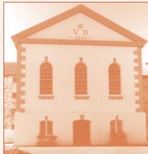
Photograph recording existing condition
