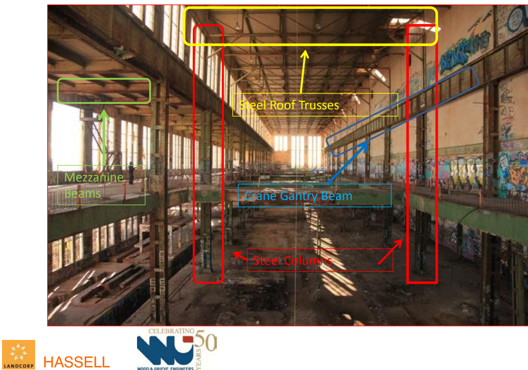
Existing Structure – Concrete (Turbine House)
