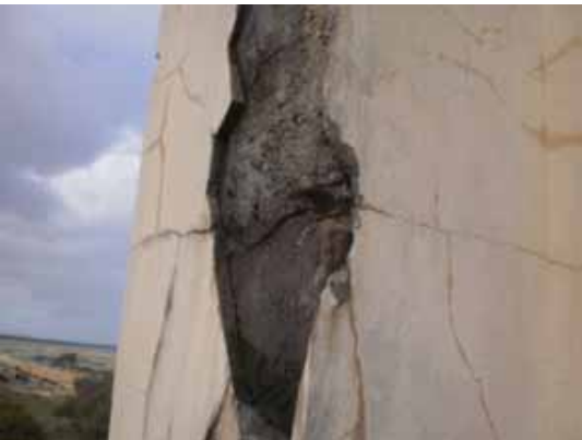
Figure 3. Example of horizontal cracking of the rendered finish on columns showing it to coincide with cold joint in the underlying concrete
