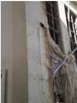
Figure 7. Example of water and corrosion staining emanating from cracks in the column
