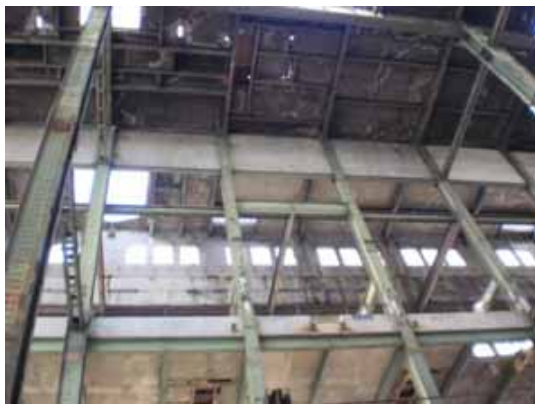
Figure 12. General view of concrete roof from the inside showing evidence of efflorescence, water ingress and areas of reinforcement corrosion and concrete spalling
