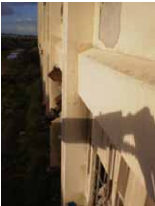
Figure 2. Typical example of cracking on columns
