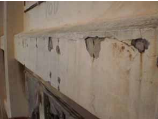
Figure 5. Example of cracking, delamination and spalling of the rendered finish on beams as well as the associated corroding metal elements embedded close to the surface
