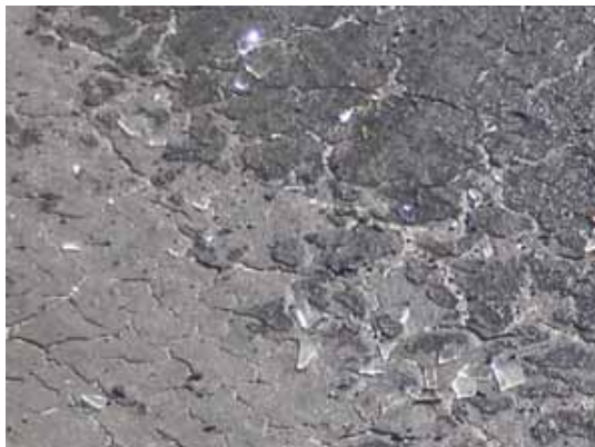
Figure 11. Typical condition of waterproofing membrane showing widespread cracking and deterioration
