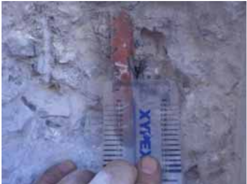
Figure 16. Width of steel flange exposed at the location with sound concrete cover
