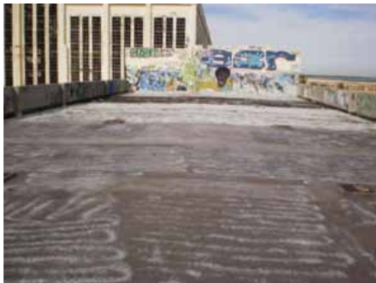
Figure 10. Typical waterproofing membrane on flat concrete roof areas
