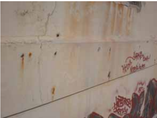
Figure 8. Example of corroded fixings or reinforcing causing small areas of concrete and render cover to spall away
