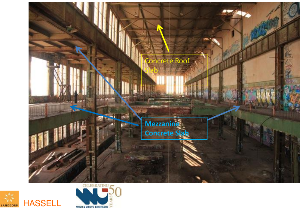
Existing Structure – Concrete (Turbine House)
