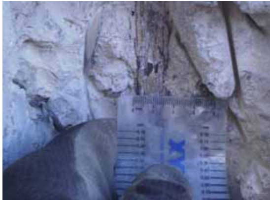
Figure 14. As found condition of steel beam at the location of a breakout coinciding with a significant crack in the concrete cover
