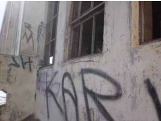
Figure 9. Example of cracking around window frames possible associated with corrosion of embedded frame fixings
