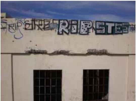
Figure 4. Concrete delamination and spalling along the bottom edge of a parapet wall exposing the corroding reinforcing steel
