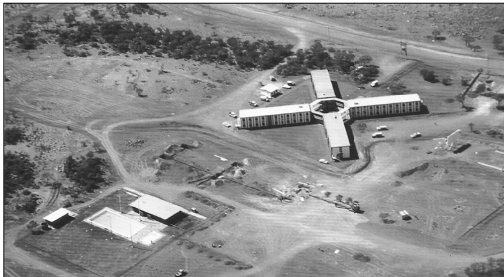
Photograph 7.1. The First Single Men's Quarters at Mt. Newman, Western Australia, 1968. 32
