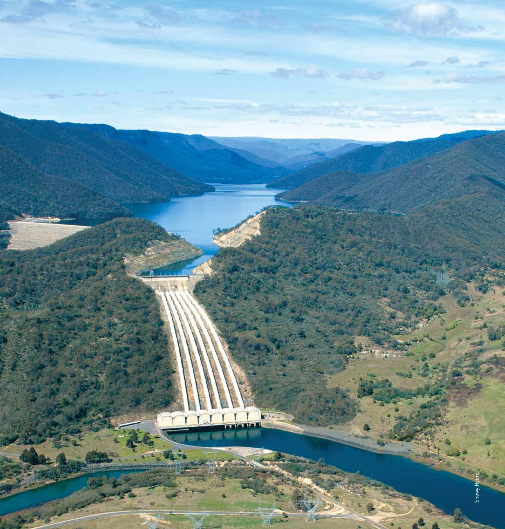
Tumut 3 power station, Snowy
